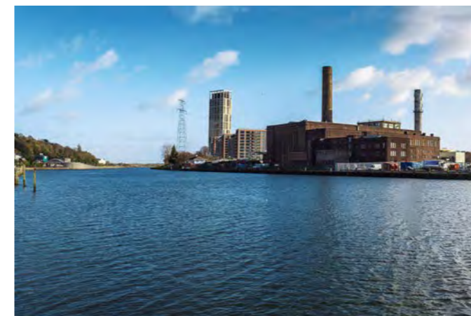
VIEW 7 Horgan's Quay
