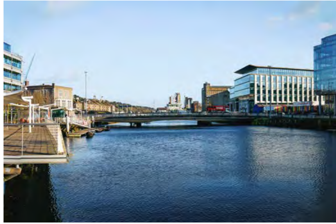
VIEW 9 Clontarf Bridge, Cork City Centre
